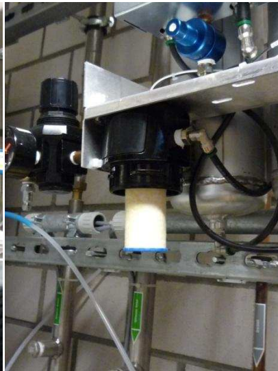
This is the inside. Need to pull it down gently.
